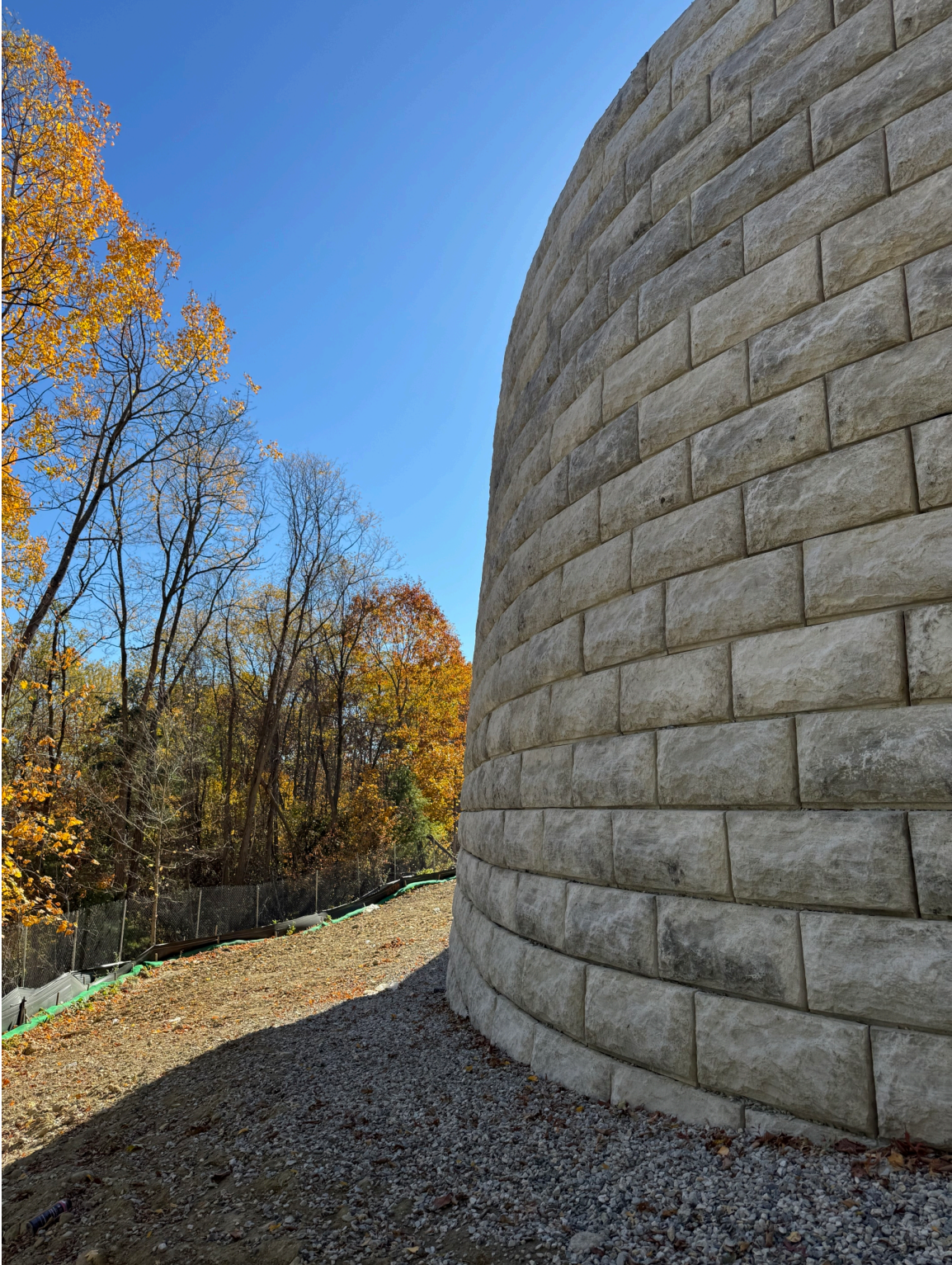
Image 1: Completed tall retaining wall at a development site
